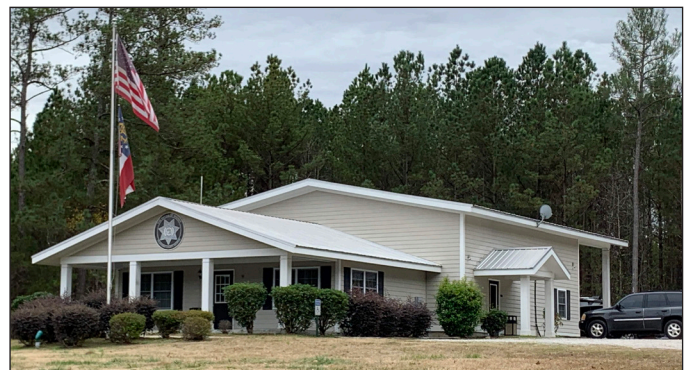
Taliaferro County Sheriff's Office
