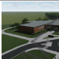
Aerial looking towards the revitalized Mu
