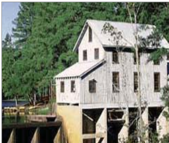
Picture 4: Water-powered grist mill at Hamburg SP
