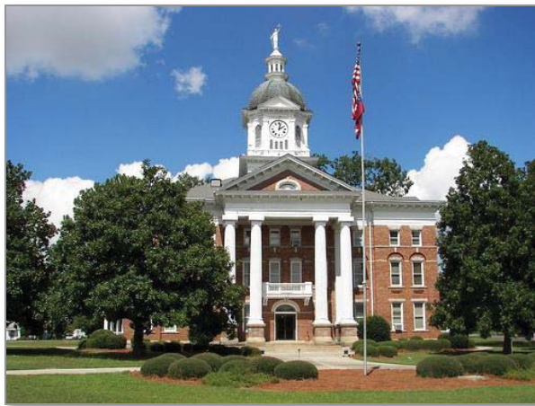
Picture 34: Jenkins County Courthouse
