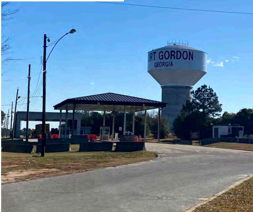
Fort Gordon Water Tower, Grovetown
