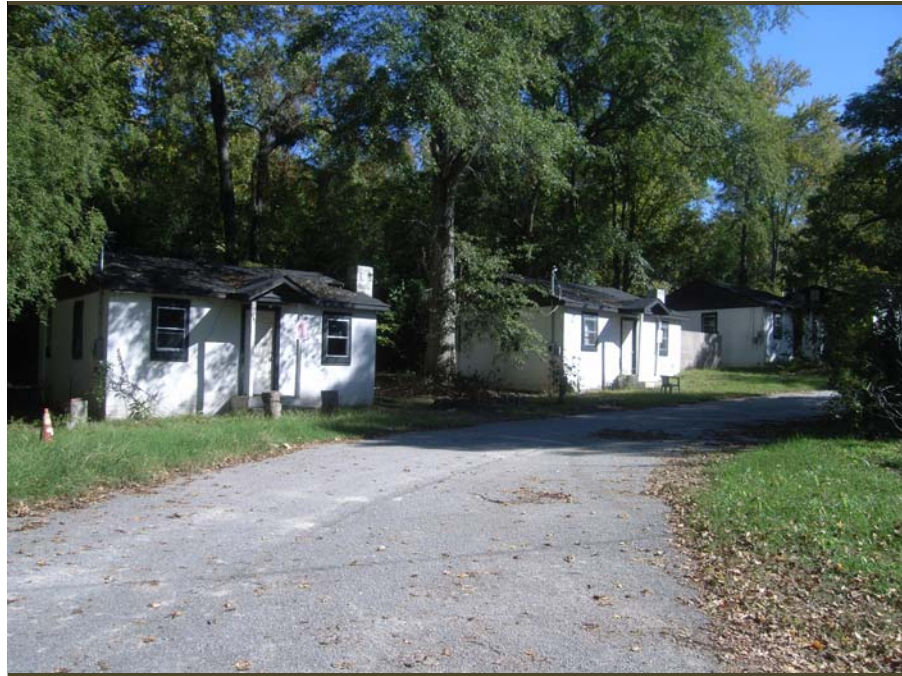
In part by suppressing surrounding property values, the “improvement” value of property containing dangerous and vacant structures provides greater liability than revenue for the city. Scenes such as these do not generate investor confidence.
