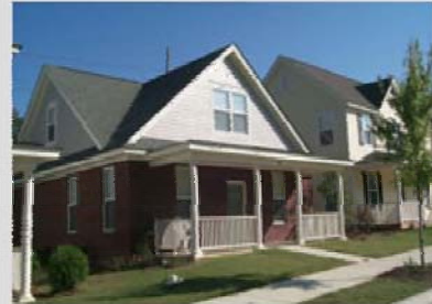
Form-based design guidelines can promote a preferred development pattern by focusing on basic building dimensions and site layout rather than decorative features and materials that can increase costs.
