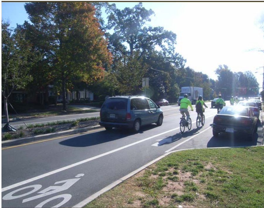
Context sensitive design: East Boulevard in Charlotte following a “road diet” from four (4) to three (3) lanes. Added bike lanes, on-street parking, landscaped medians, pedestrian “refuge islands. Carries over 21,000 AADT—81 percent more motor vehicles than Robinson Avenue.
