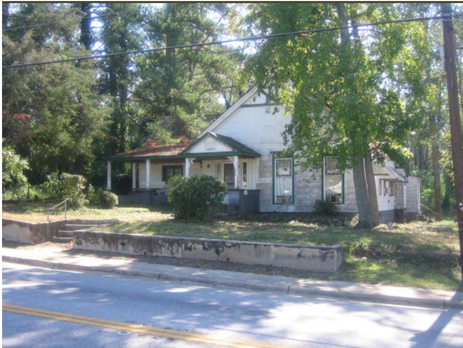
Many residential properties still flank Robinson Avenue. Grovetown will need to determine how residential rehabilitation is incorporated into a new “downtown.”
