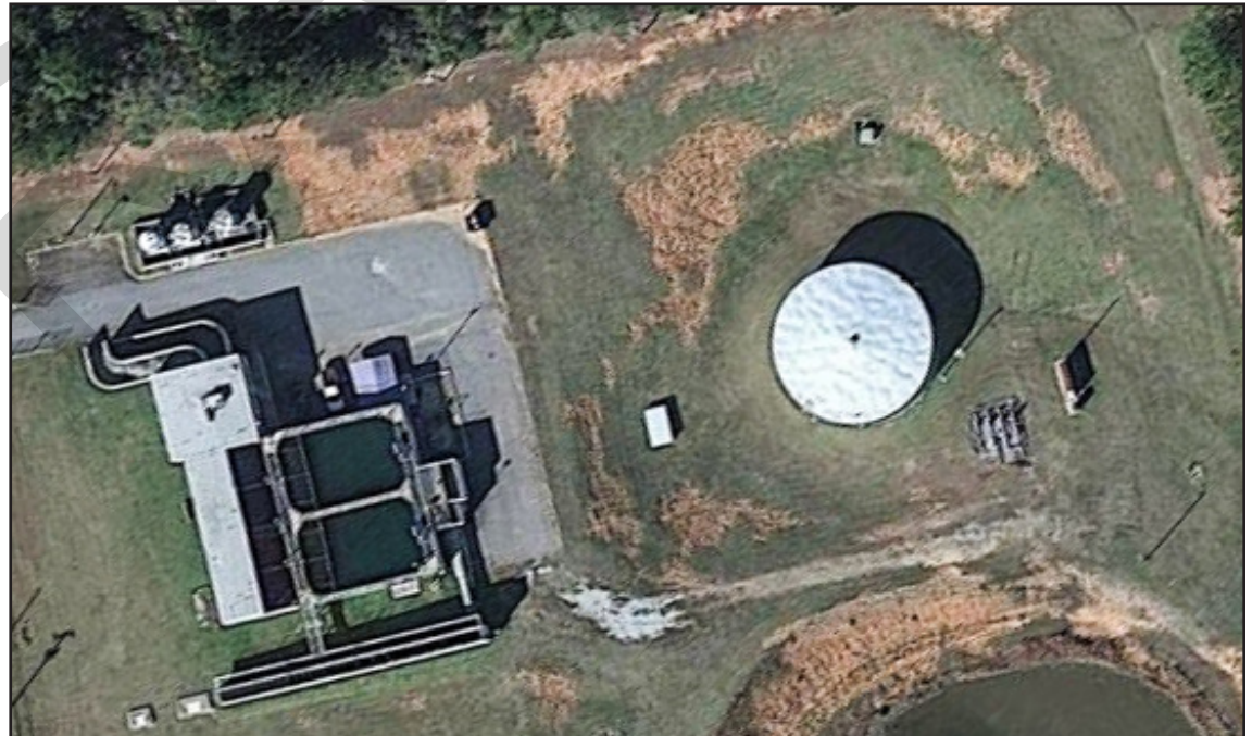
The Aonia Water Treatment Facility opened in 1978 and provided a capacity of 2 million gallons per day.
