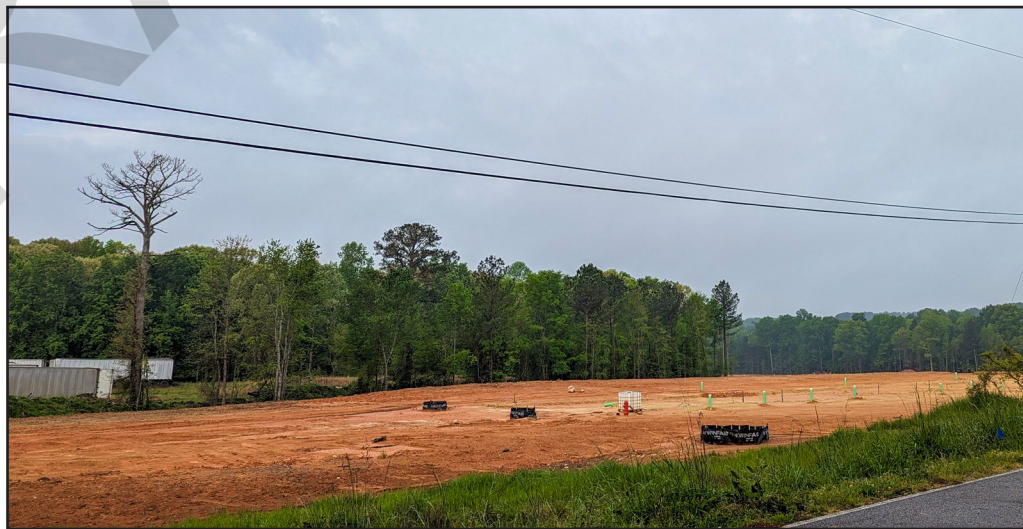
A new subdivision is under construction on Ashley Drive.
