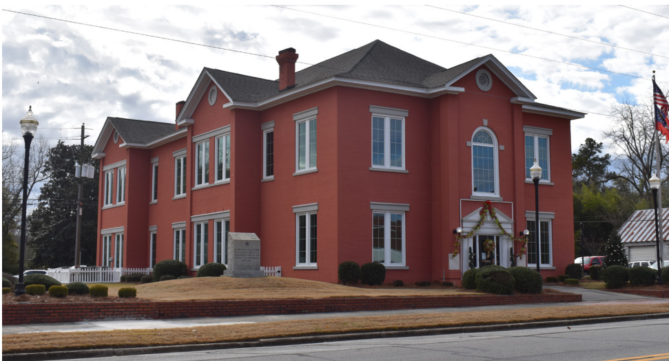
1) Glascok County Courthouse, Listed in the statewide NR thematic nomination for courthouses in Georgia as a contributing building.
