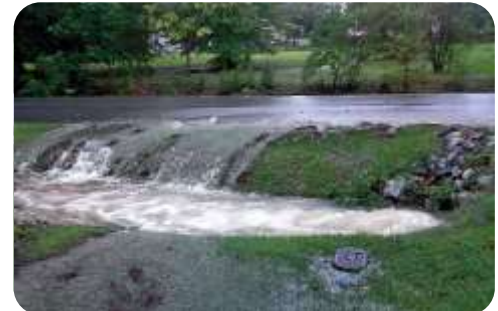
2013 CDBG Funds will correct this kind of flooding in the Town of Dearing
