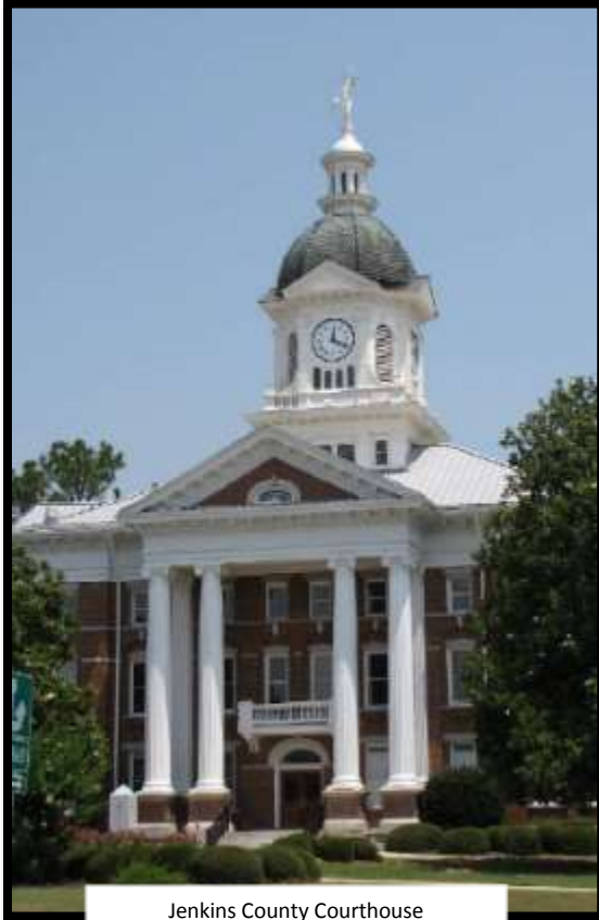
Jenkins County Courthouse
