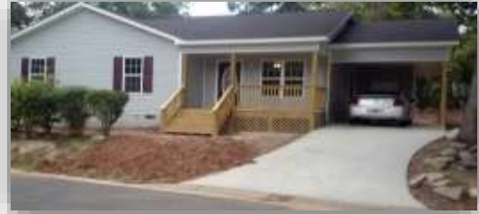
Sandersville 09 CHIP House Reconstruction
