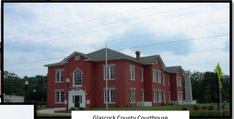
Glascock County Courthouse
